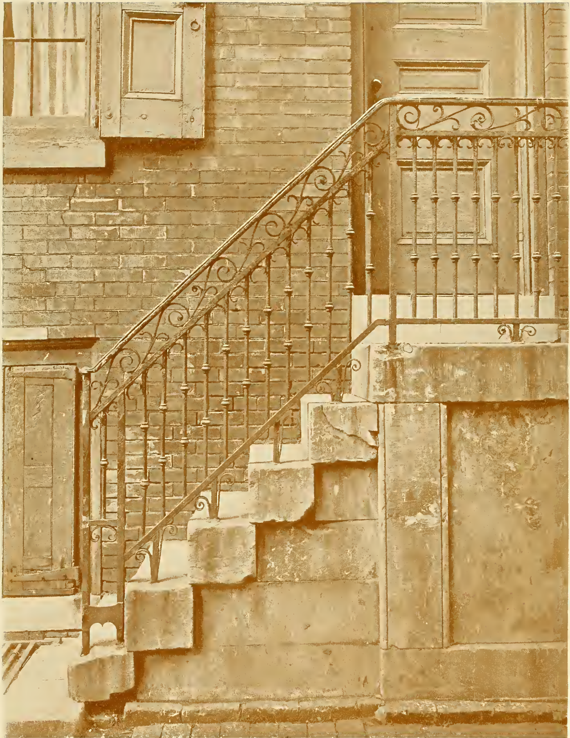
BALUSTRADE, SECOND AND LAGRANGE STREETS Philadelphia
